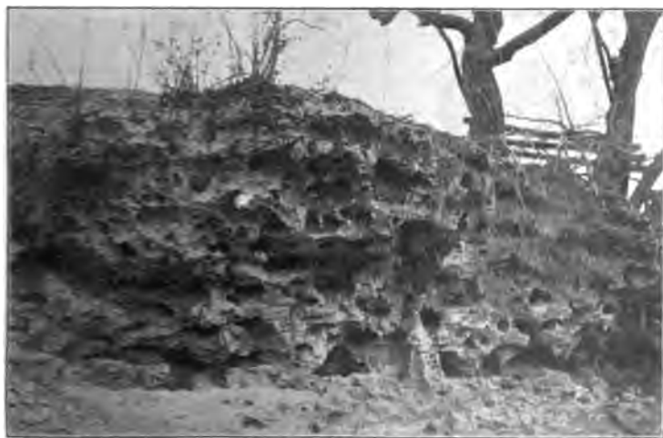
FIG. 14. Honeycombed Limestone, Iowa
